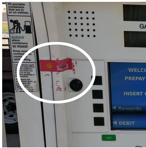
(a) This pump is normal. It has a single, unbroken, correctly-placed seal.
