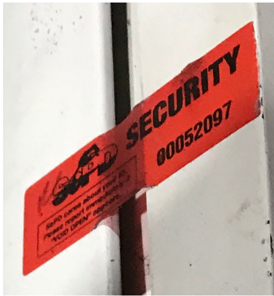
Fig. 7: This style of seal is used throughout a municipality. In order to identify whether the correct seal is being used, consumers must be aware of the type of seal expected to be present.
